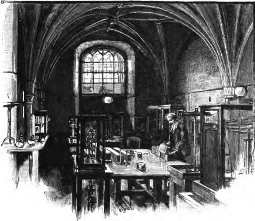
Fig. 29.—BASEMENT OF THE JEWEL TOWER NOW USED AS A BALANCE ROOM.
